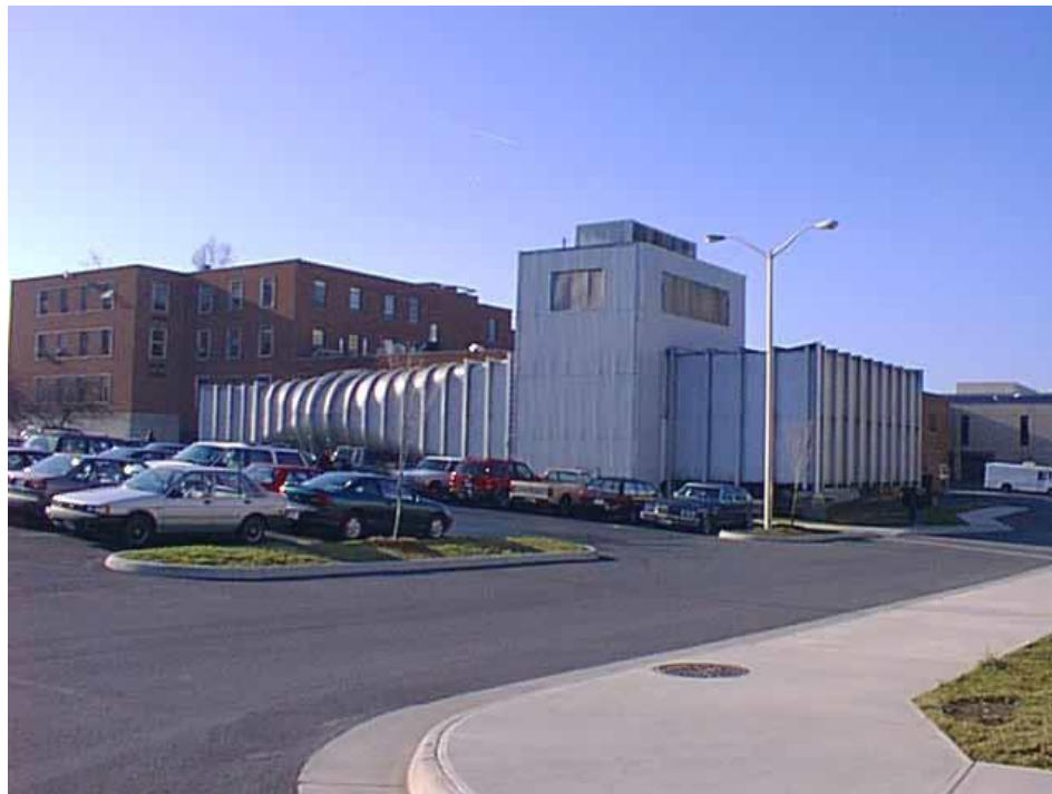
Figure 2.4 The Virginia Tech Stability Wind Tunnel. The Air Exchange Tower is Clearly Visible. The Tunnel Fan and Motor Assembly is Located Inside the Tunnel to the Left of the Air Exchanger. (Photo by Aerospace and Ocean Engineering Department, VPI & SU – Used under fair use, 2013).
