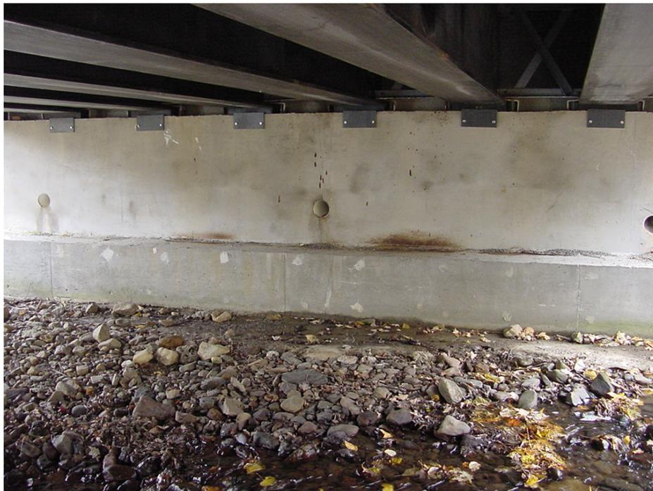
**Figure 6-6.** Extent of river stone pile-up at east abutment during Fall 2003 inspection of the Route 601 Bridge.
