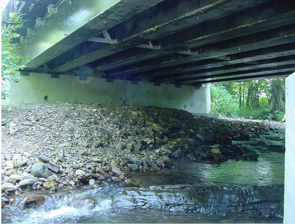
**Figure 6-7.** Extent of river stone pile-up at east abutment during Spring 2004 inspection of the Route 601 Bridge.
