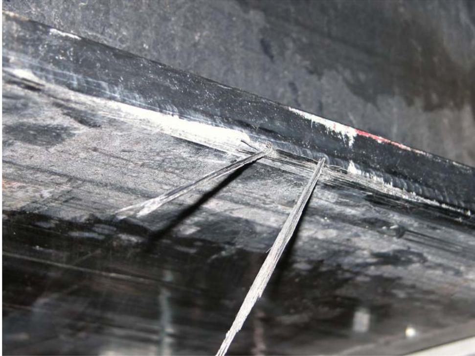
**Figure 6-3.** Matrix resin material splintering off from Girder 5 of the Route 601 Bridge (courtesy of Strongwell Corp).
