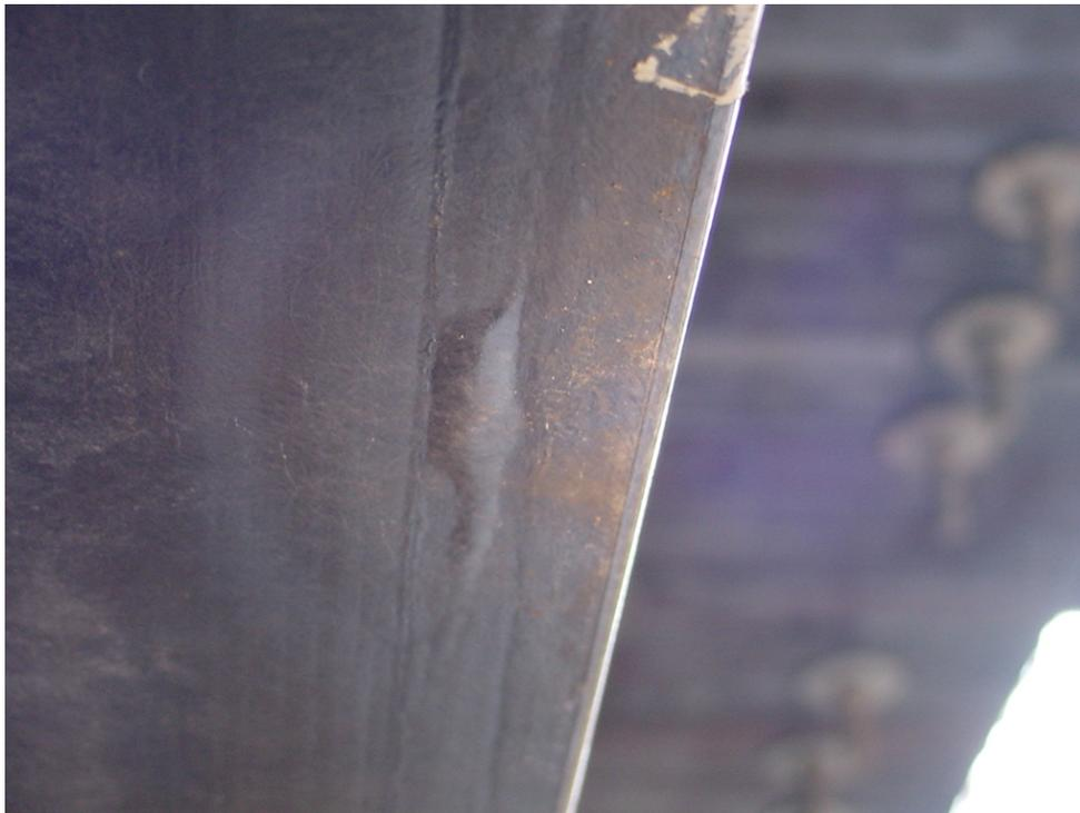
**Figure 6-4.** Typical blister on the surface of the bottom flange in an exterior girder for the Route 601 Bridge.
