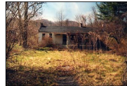
(Fig. 4.12) Cottage in ruin – Warm Springs, VA
