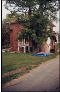
(Fig. 4.16) Brick Cottage under Repair Old Sweet Springs, WV
