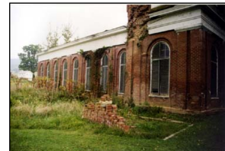
(Fig. 4.44) Exterior of bath house – Old Sweet Springs, WV
