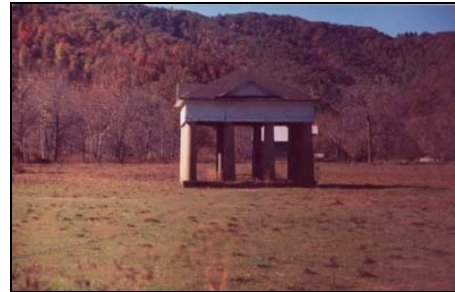
(Fig. 4.35) Spring House - Blue Sulphur Springs, WV
