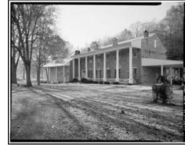
(Fig. 3.12) Salt Sulphur Springs, Main Building, NORTHEAST FRONT (Library of Congress) Prints and Photographs Division HABS WVA,32-SALSU,1A-1
