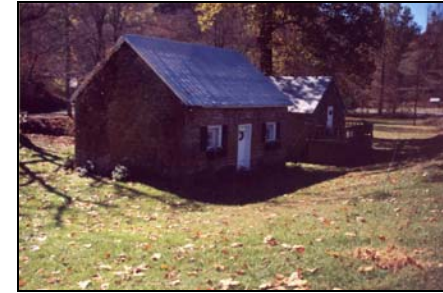
(Fig. 4.33) Stone Bath Houses - Salt Sulphur Springs, WV
