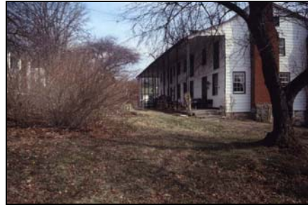
(Fig. 4.18) Range with Portico at Warm Springs, VA
