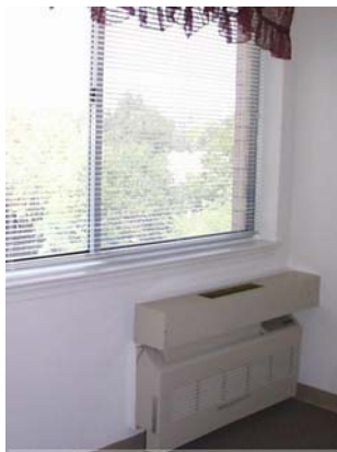
Figure 18. Facility's windows with ledges.
