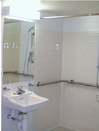
Roll-under sink, tilted mirror and wrap-around grab bar in shower
