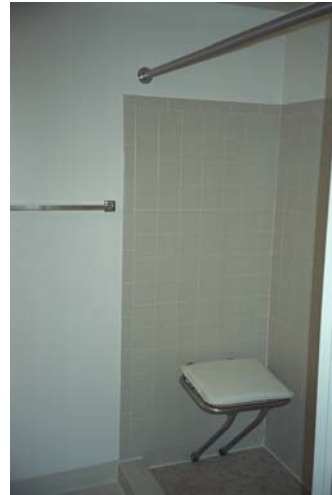
The seat is permanently attached to the wall, but no grab bars.
