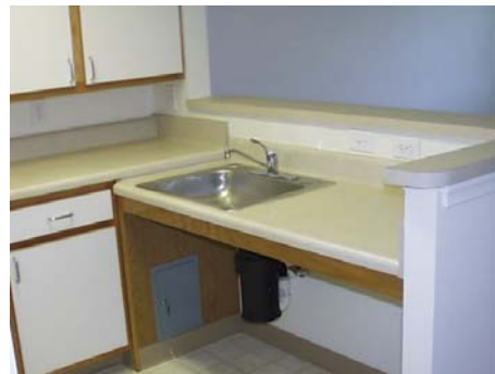
Roll-under sink & counter, open to living room.
