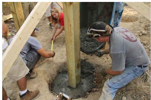
Students installing posts for the arbor
