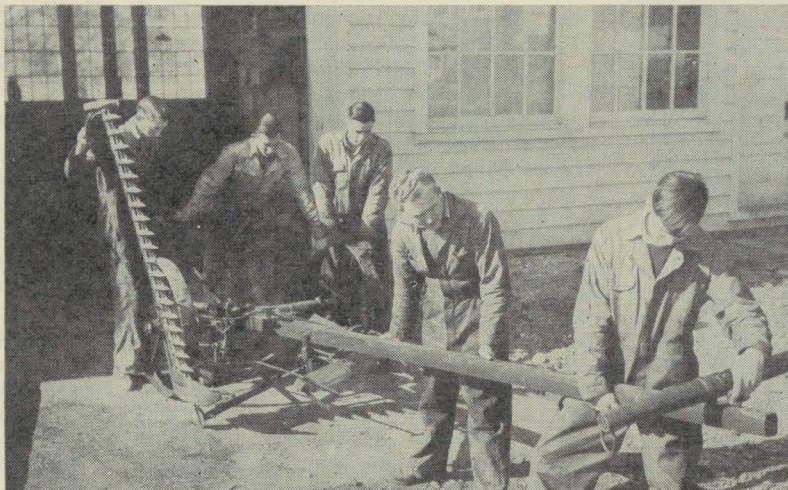
Rustburg High School Repair Program—Mower Ready for Delivery
