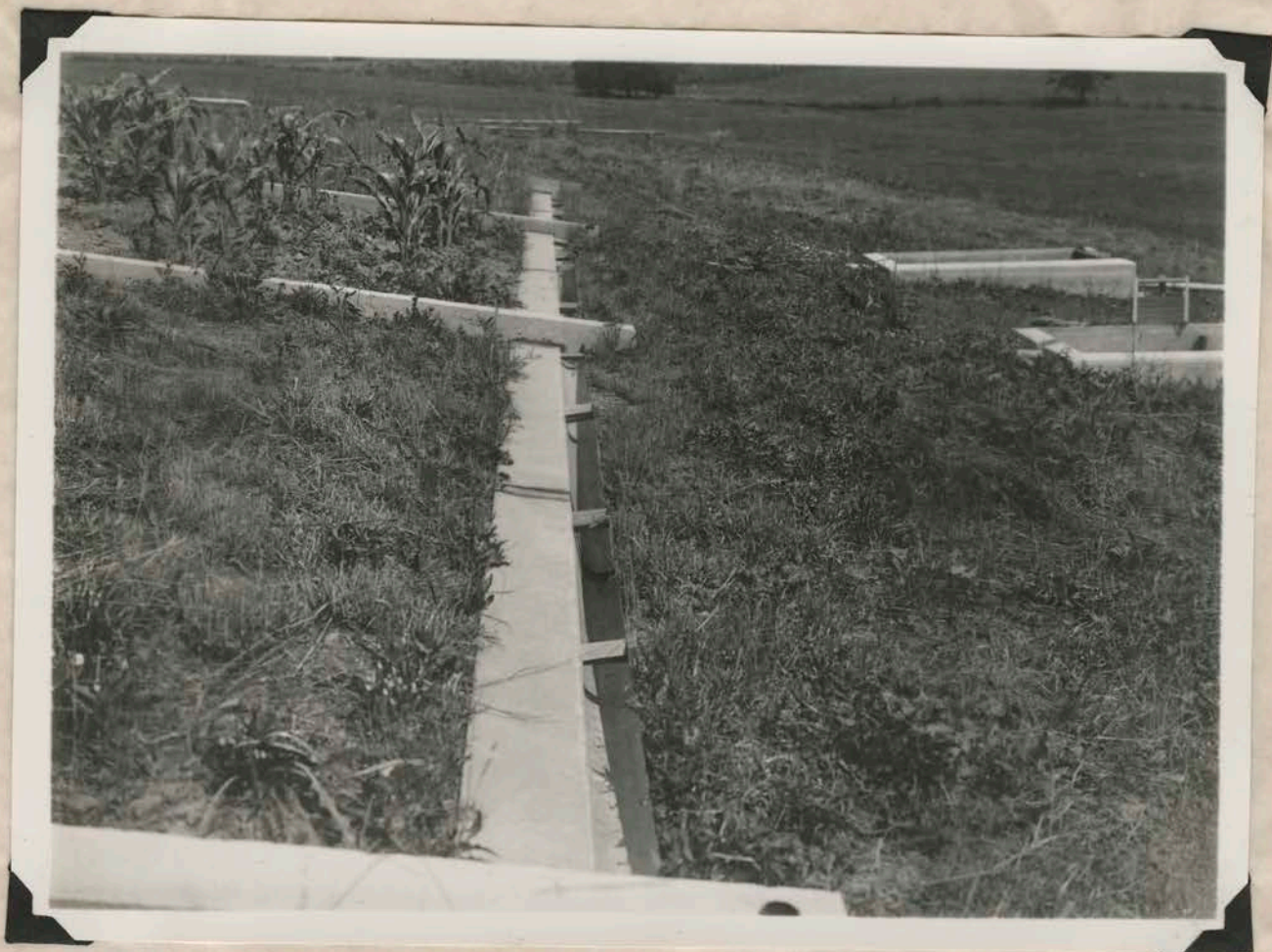
This picture shows some detail of the catchment troughs which are placed across the lower side of each plot. The runoff is conducted from these troughs through a 3" galvanized rain pipe into the concrete catchment tank shown in the picture on the following page. There is a "lip" on the up-hill side of these troughs which is forced vertically into the soil one foot.
