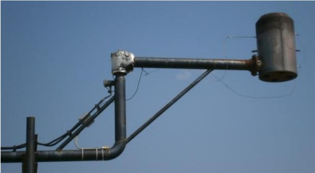
**Figure 2.6. Flare for burning excess biogas.**
