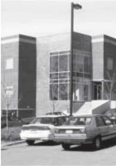
Stair Enclosure at 712 N. Main Street
