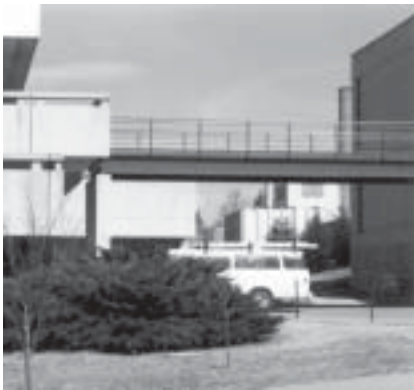
Whittemore Pedestrian Bridge
