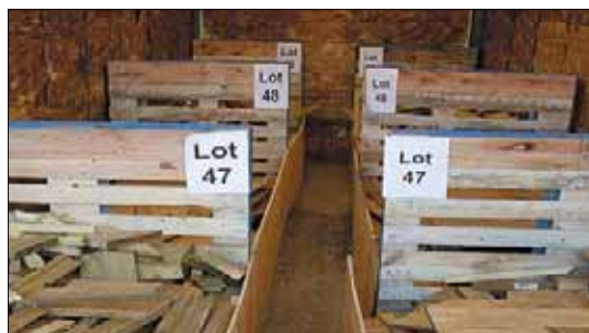
Recovered materials are sorted and stored in trailers at the construction site.
