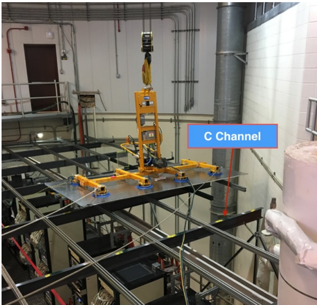
Figure 17. MicroBooNE top plane support structure and C Channel. The roof crane and rigging system is placing one module in position.
