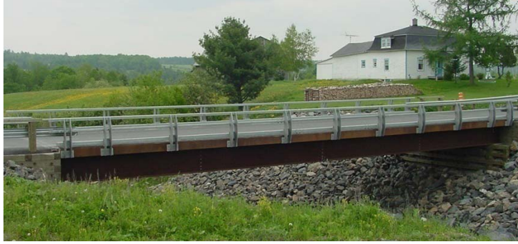
Figure 4. Shenley Bridge, Quebec, Canada
