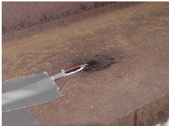
Figure 13. Strain Gauge Mounted on Girder
