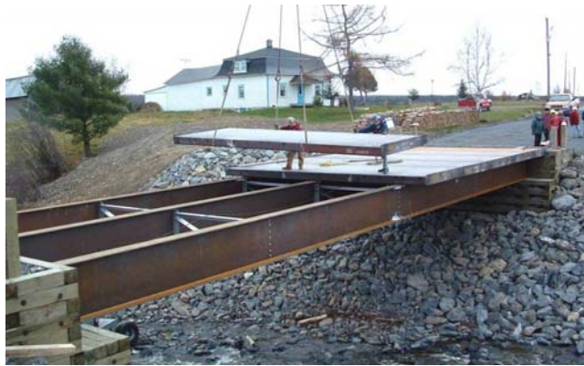
a) Deck panel installation
