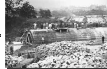
Figure 2. Wingohocking Creek Sewer under construction. Philadelphia. 1909.
