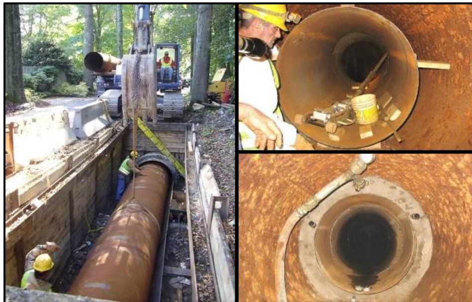
Figure 3-26. Segmental Sliplining Operations (Authority, 2009)
