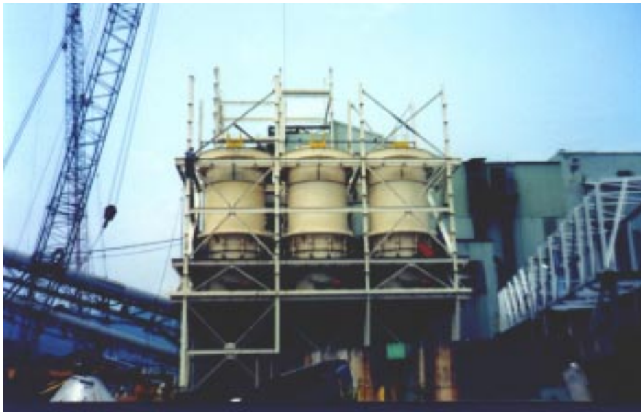
Figure 3-19. Full-scale 4-meter diameter column installation at the Lady Dunn Preparation Plant.
