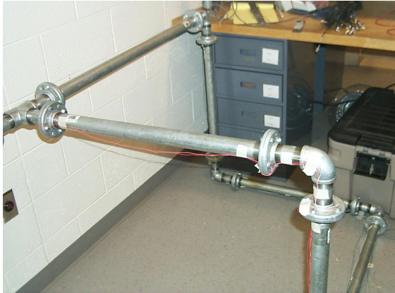
Figure 2.9 Portion of pipeline structure
