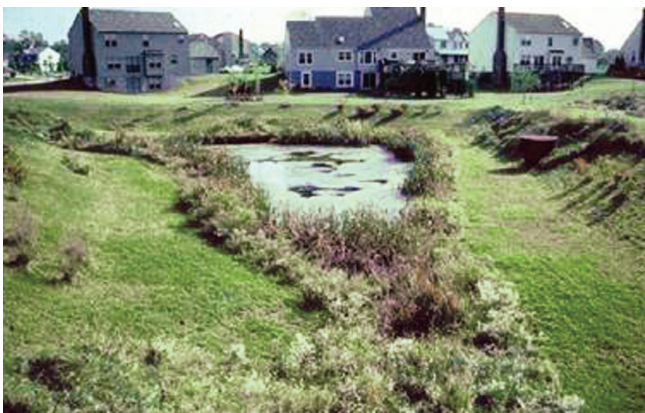
Figure 1. Extended detention pond during wet period (VA-DCR 2011).
