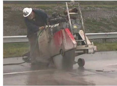
Figure 4-1 - Saw-cutting of existing pavement prior to removal
