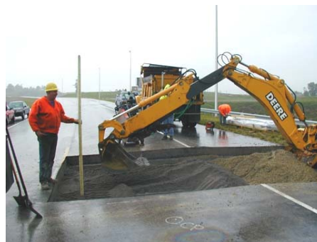
Figure 4-3 - Leveling of the excavated pit
