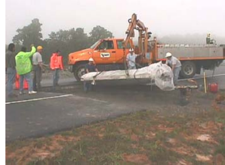
Figure 4-5 - Initial placement of the scale by VDOT boom truck
