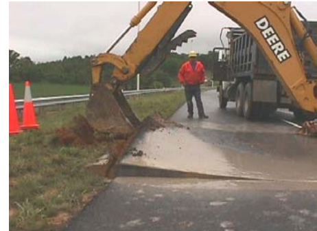
Figure 4-2 - Removal of existing pavement by backhoe
