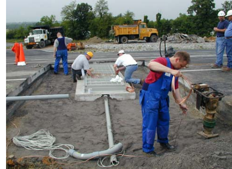
Figure 4-6 - Installation of conduit and grounding wires
