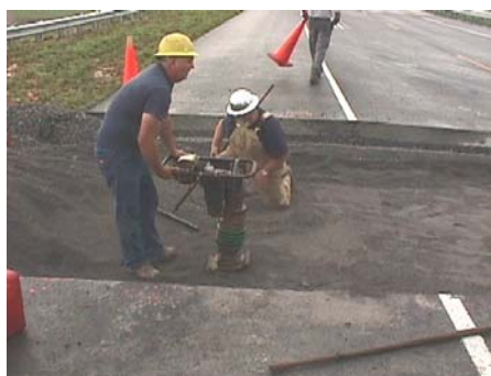
Figure 4-4 - Compaction of the base material prior to placement of the scale
