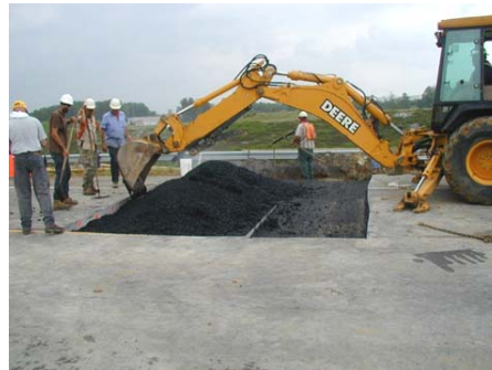
Figure 4-8 - Placement of first lift of BM-2 layer
