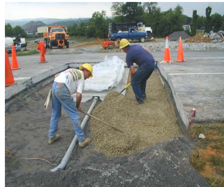
Figure 4-7 - Placement of granular base material over conduit
