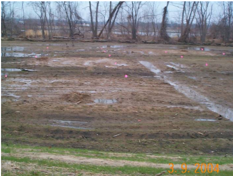
Figure 12. Site after the application of soil amendments and installation of microtopography in March of 2004. Photograph by Lee Daniels, used with permission.
