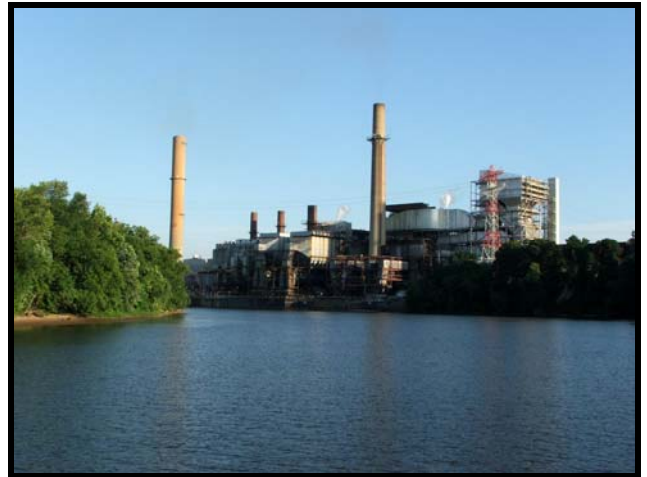
Dominion's Chesterfield Power Station (Chesterfield County), June 22, 2007.
