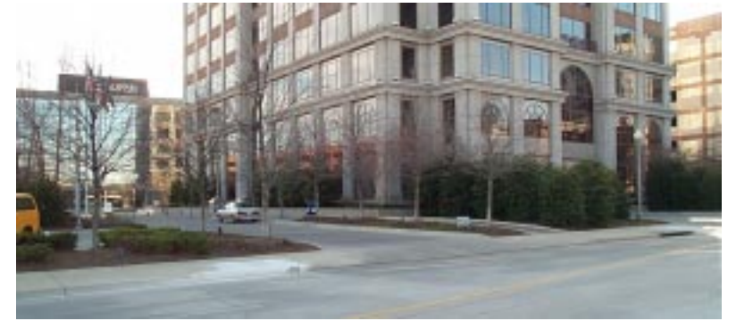
Parking lot to Norfolk Southern Building (26)
