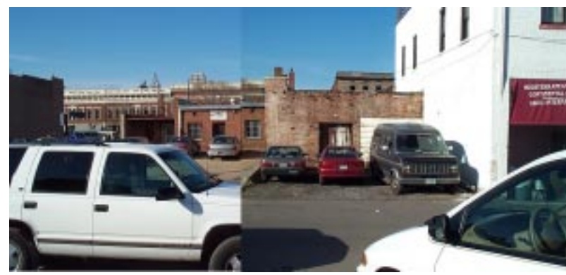
Condition of buildings facing parking lot (16)
