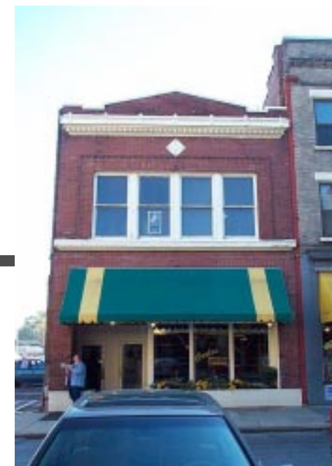
Carlos' Brazilian Restaurant (right of site) (20)
