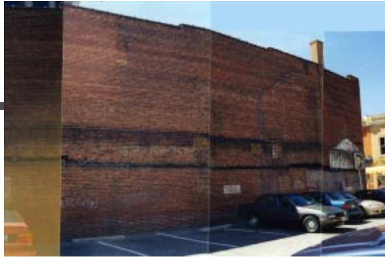
Side view of Carlos' showing condition of brick (21)
