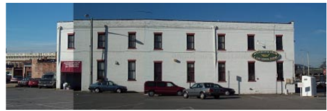
Condition of restaurant facing parking lot (17)
