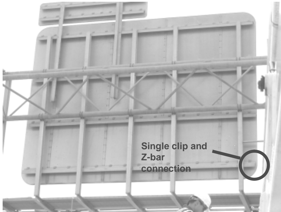
Figure 9. Sign Connected to Support.
