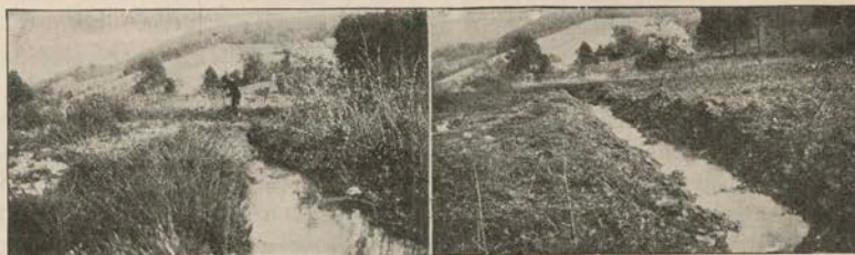
Fig. 11—View of Ditch Before and After Cleaning Out by Use of Explosives
