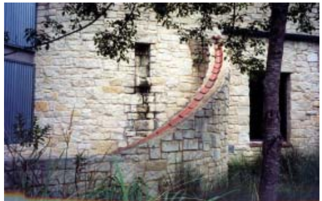
Examples from the Lady Bird Johnson Wildflower Center in Austin, TX showing how rooftop rain water can be harvested.
