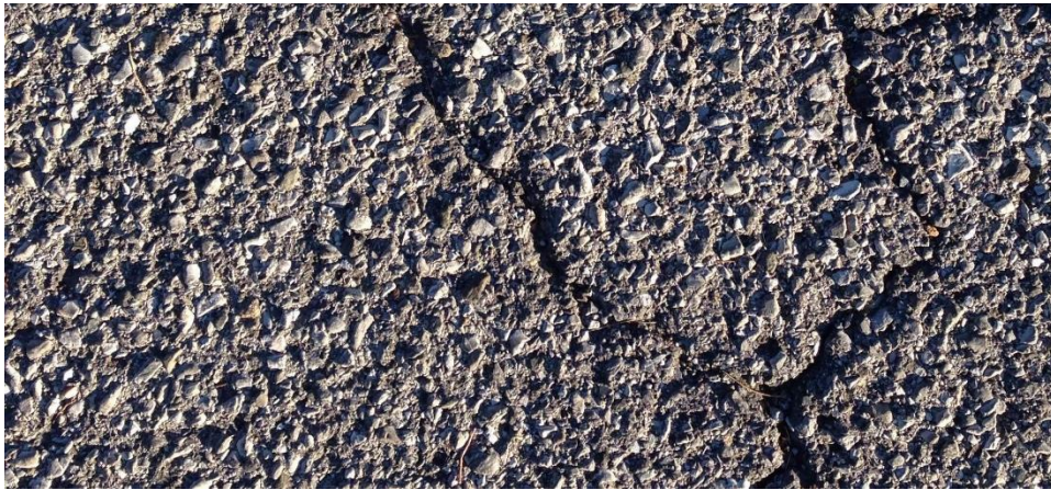
Figure 4.1: Example of micro-shadows cast by low sun angle and significant surface texture caused by pavement erosion.
