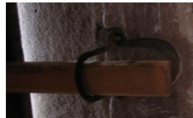
Figure 3.14. Door lock of the Yin Yu Tang house. Photograph by the author, courtesy of the Peabody Essex Museum.
