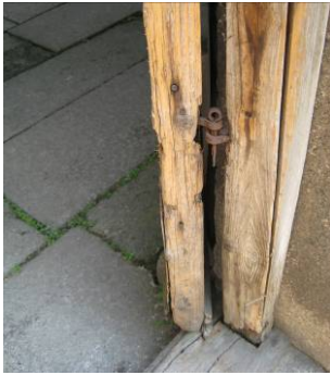
Figure 3.16. Pin and hook hinge in a Huizhou house. Photograph by the author.
