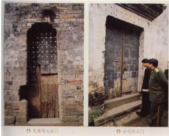
Figure 3.31. The fireproofing doors in Huizhou, Li Jun, Huizhou gu min ju tan you , 2003.
