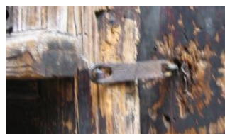
Figure 3.13, Yin Yu Tang door lock using the pin-and-hook mechanism. Photograph by the author, courtesy of the Peabody Essex Museum.
