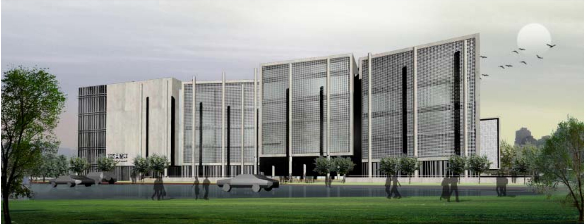
GENERAL VIEW ACROSS THE STREET
