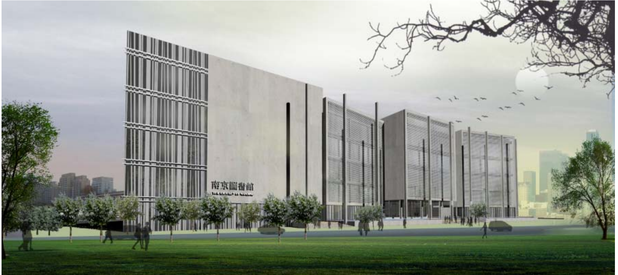
GENERAL VIEW ACROSS THE STREET
