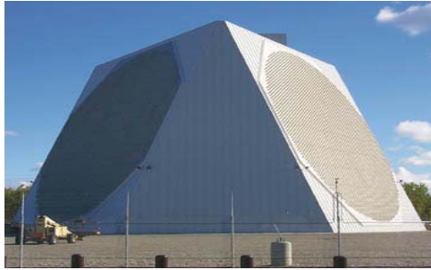
Figure 2.2: 90-foot diameter planar phased array - Alaska - Clear Radar Upgrade program (Photo courtesy of Alaska District)
