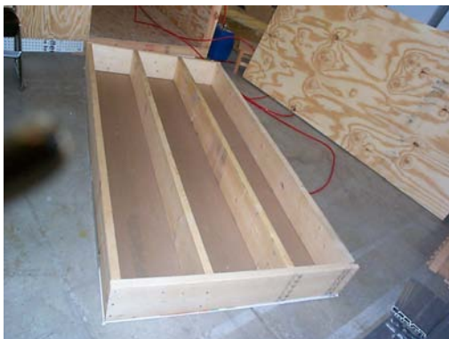
Figure 4-3-2-4a: RAUPANEL 8" o.c w/o insulation Construction (1)
