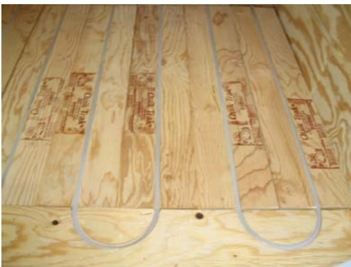
Figure 4-3-2-6a: QuickTrak 7" o.c Construction (1)
