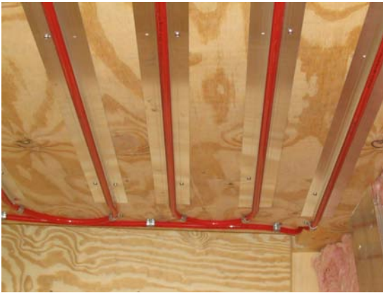
Figure 4-3-2-12a: Joist Space 8" o.c w/ plates Construction (1)
