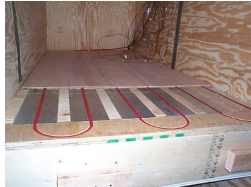
Figure 4-3-2-4b: RAUPANEL 8" o.c w/o insulation Construction (2)
