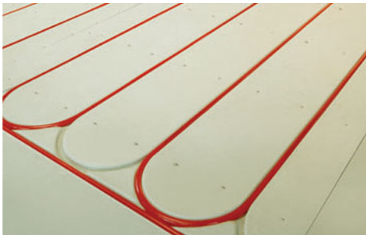
Figure 2-5-5: Warmboard Installation
