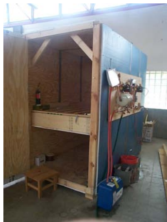
Figure 4-3-1-4a: Hot Water Circulation Loop (front side view)
