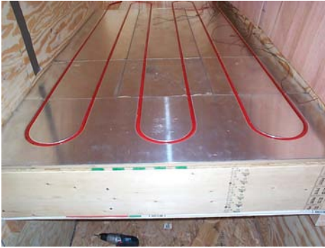
Figure 4-3-2-5a: Thermalboard 8" o.c Construction (1)
