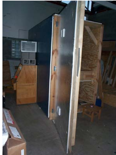
Figure 4-3-1-1g: Test Chamber Construction (4)
