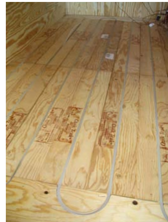
Figure 4-3-2-6b: QuickTrak 7" o.c Construction (2)
