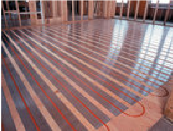
Figure 2-5-6: RAUPANEL Radiant Floor Installation
