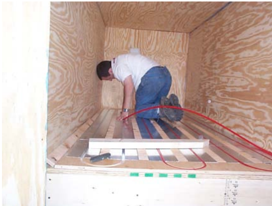
Figure 4-3-2-3a: RAUPANEL 8" o.c w/ insulation Construction (1)
