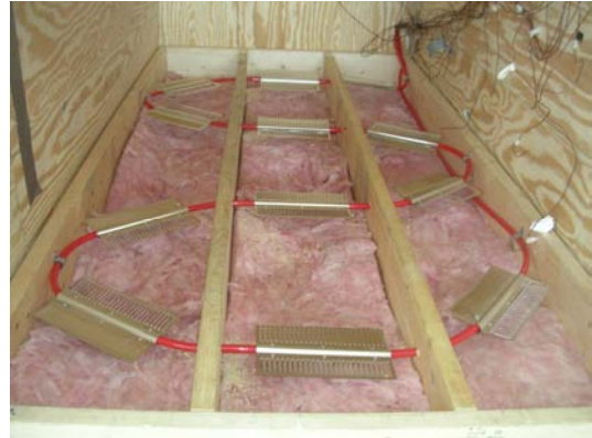
Figure 4-3-2-10b: UltraFin Construction (2)
