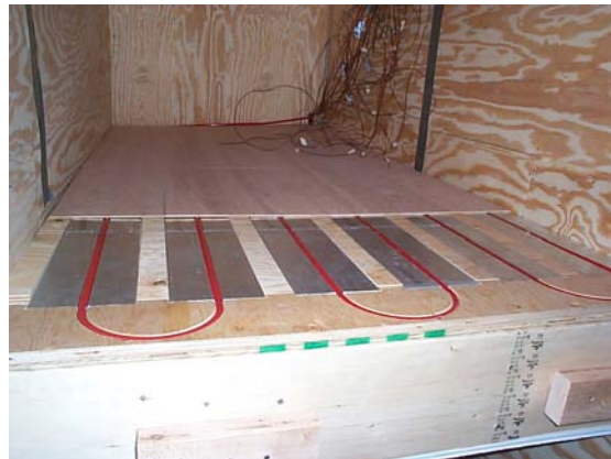
Figure 4-3-2-3b: RAUPANEL 8" o.c w/ insulation Construction (2)
