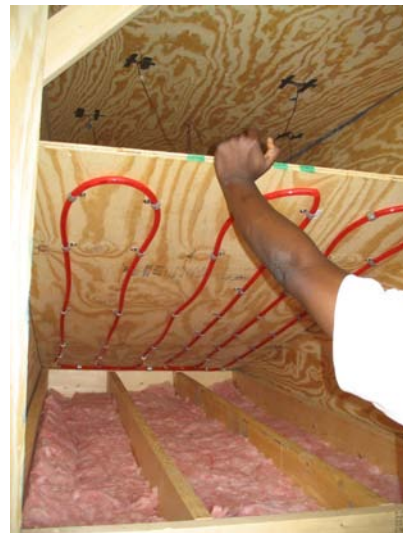
Figure 4-3-2-11b: Joist Space 8" o.c w/o plates Construction (2)
