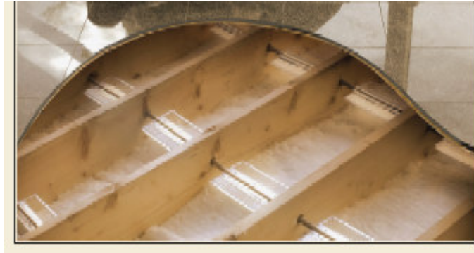
Figure 2-5-2: Ultra-fin Installation
