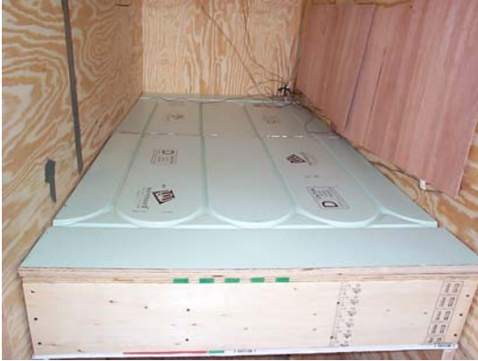
Figure 4-3-2-7a: Warmboard 12" o.c Construction (1)
