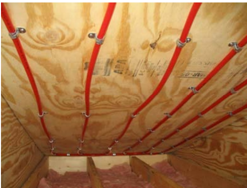
Figure 4-3-2-11a: Joist Space 8" o.c w/o plates Construction (1)
