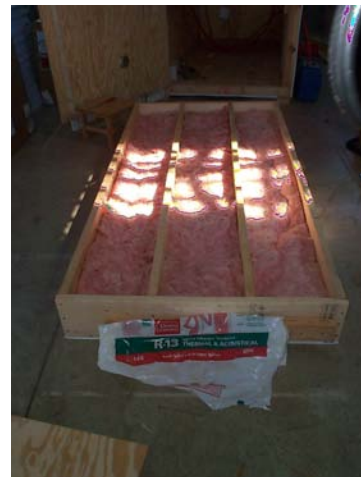
Figure 4-3-1-2c: Radiant Floor Test Device Construction (2)
