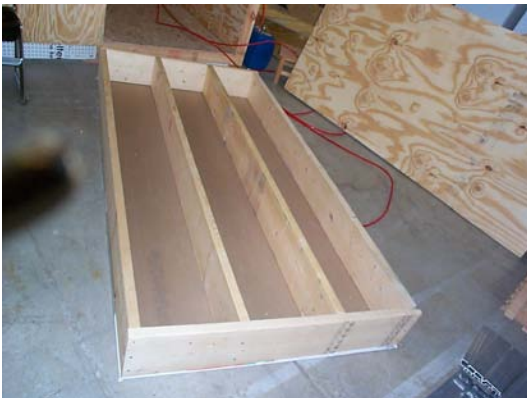
Figure 4-3-2-2a: RAUPANEL 6" o.c w/o insulation Construction (1)
