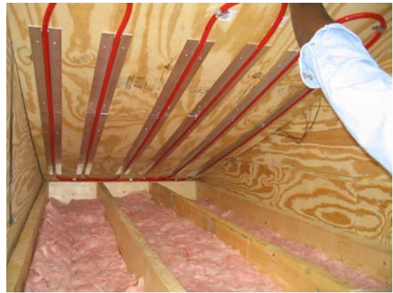
Figure 4-3-2-12b: Joist Space 8" o.c w/ plates Construction (2)
