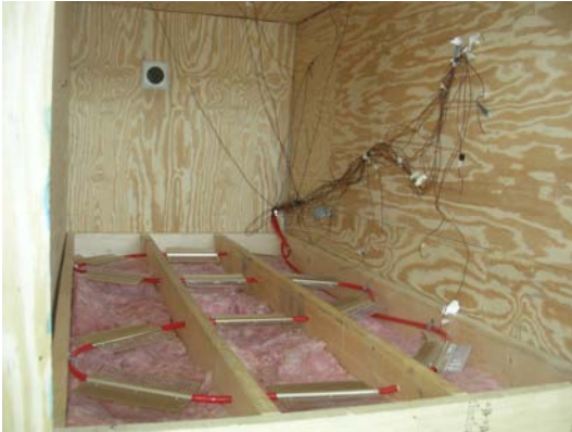
Figure 4-3-2-10a: UltraFin Construction (1)
