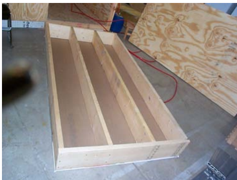
Figure 4-3-1-2b: Radiant Floor Test Device Construction (1)
