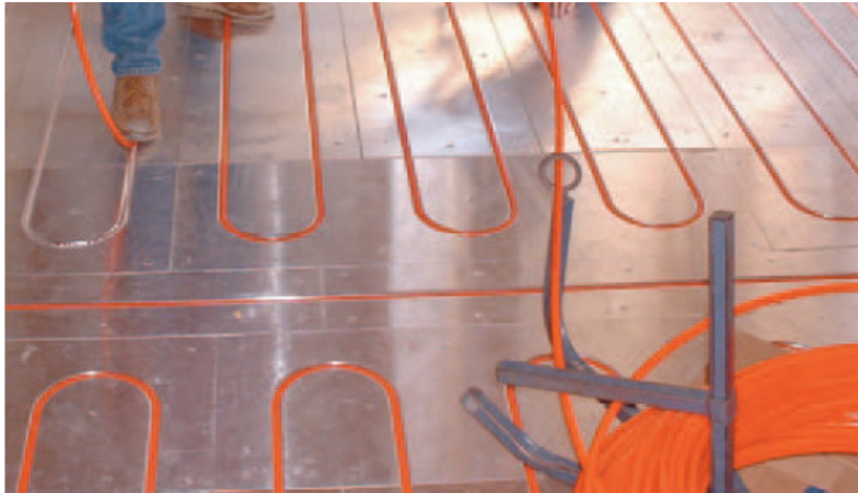
Figure 2-5-4: Thermalboard Radiant Floor Installation
