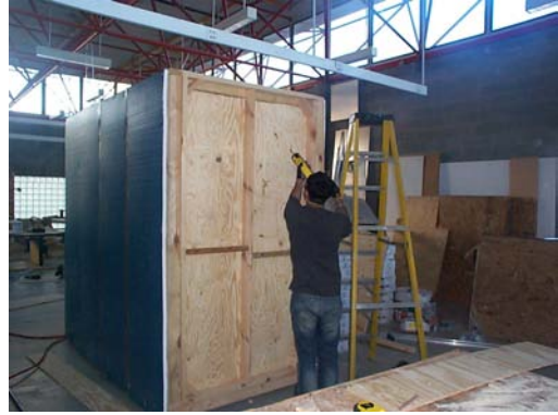
Figure 4-3-1-1e: Test Chamber Construction (2)
