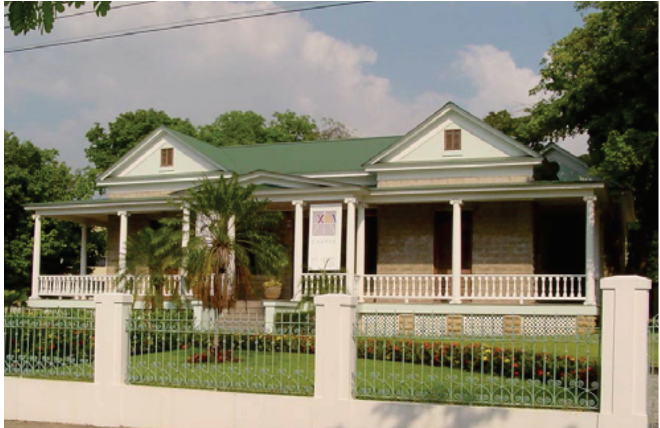
Existing North West Elevation, Gonzalez Cuyar House
