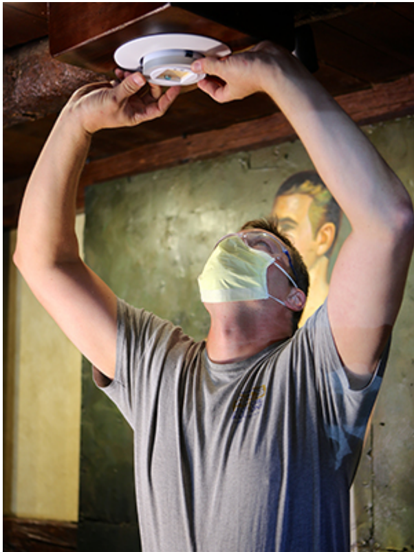
Photo: Installation of Heathe Lighting.
