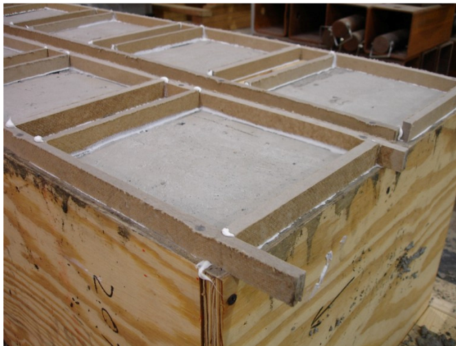
Figure 3-4: Homasote Board attached to formwork to contain epoxy layer
