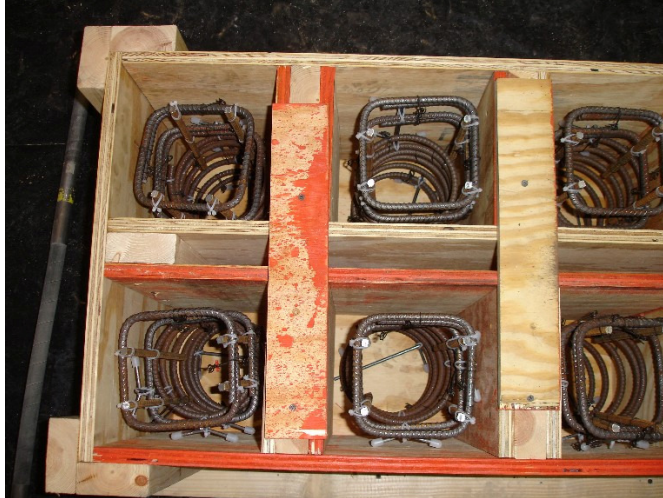
Figure 3-3: Reinforcing cages in the formwork
