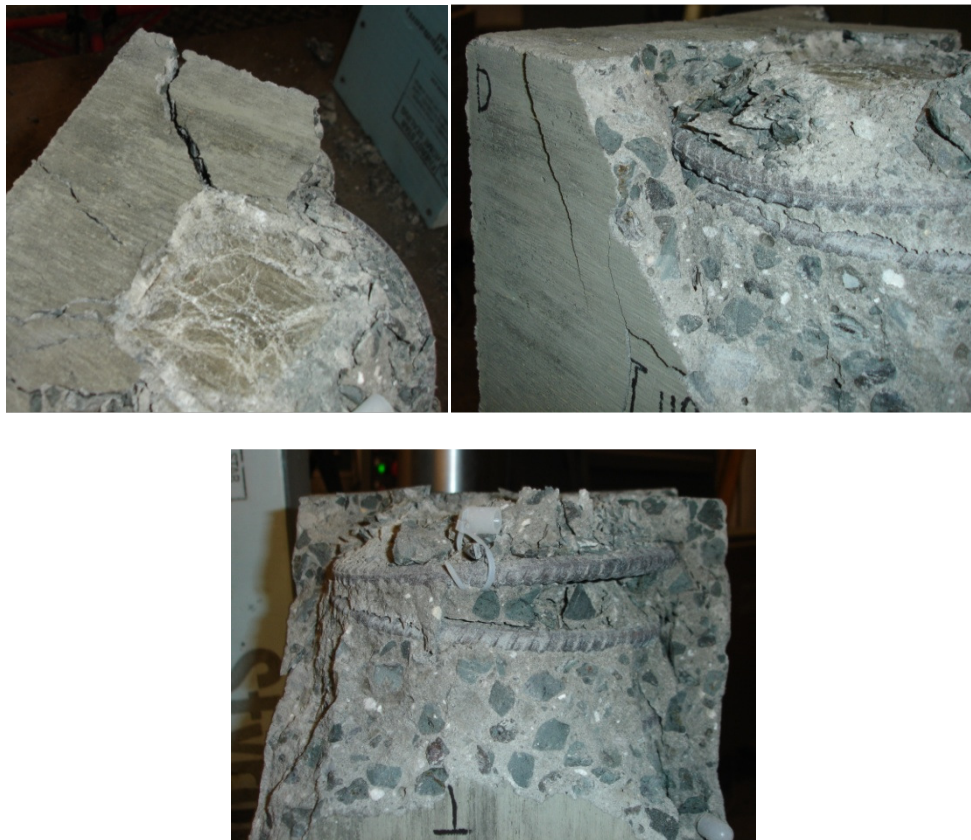
Figure 4-14: Detail of Concrete Beneath the Bearing Plate
