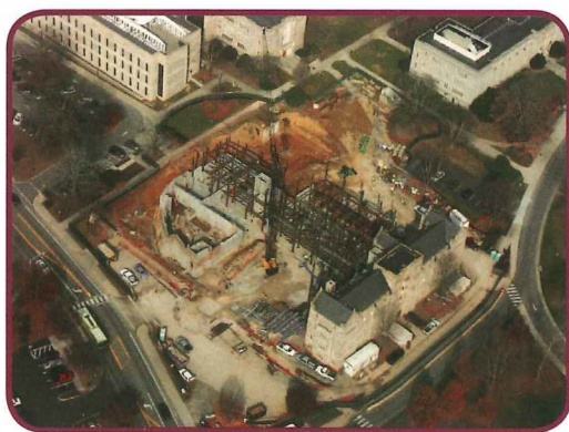
Aerial view of Davidson construction
