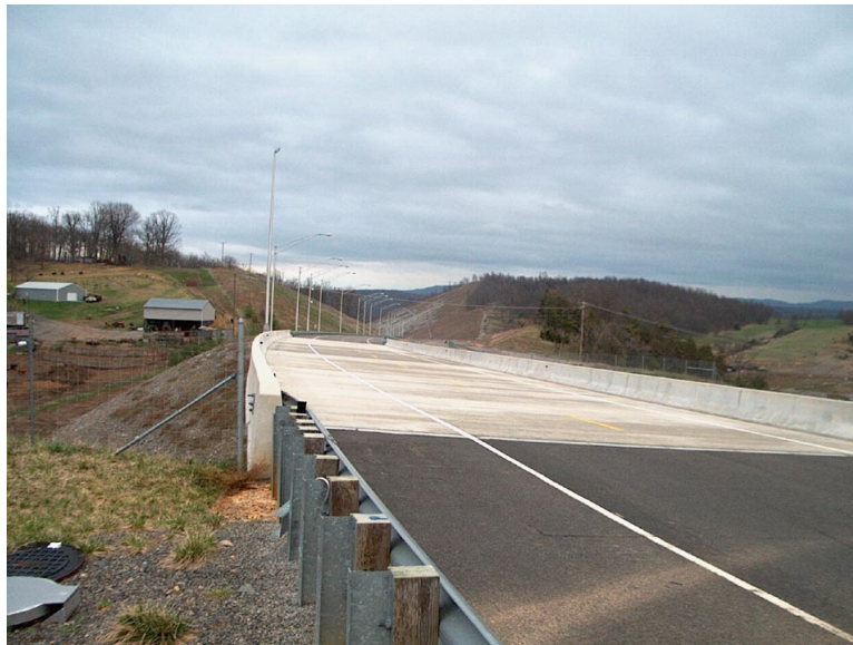
Figure 3. 8: A View from Second Wireless Node along The Road
