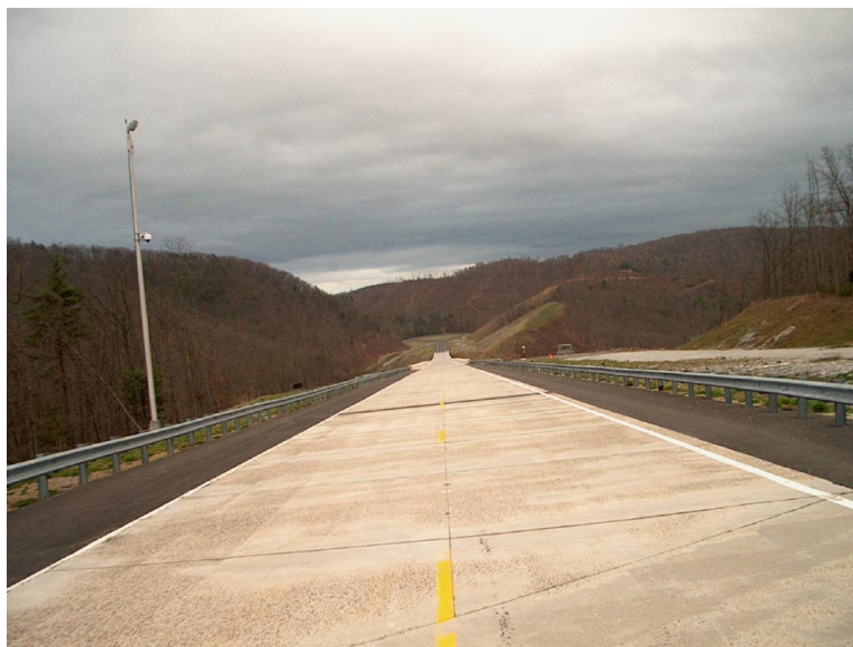
Figure 3. 10: A View from Last Wireless Node on The Road
