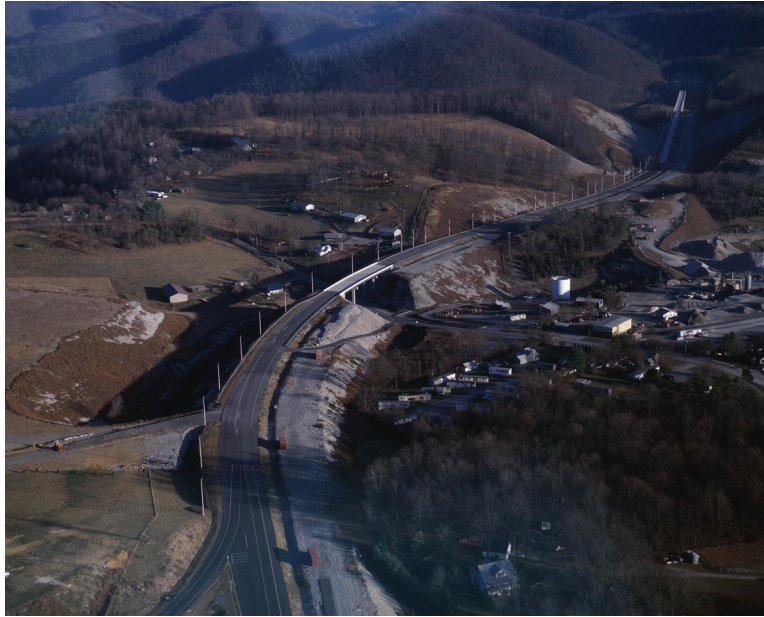
Figure 3. 2: An Aerial View of The Smart Road
