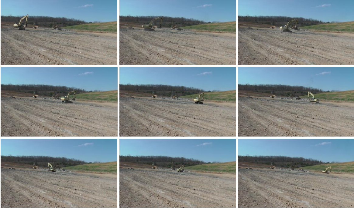
Figure 2.8: Sample video frames demonstrating the excavator's path
