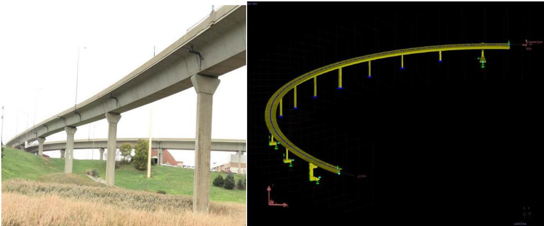
Figure 2.4: Illinois Tollway bridge in Finite Element Model (Ciorba Group, public domain)
