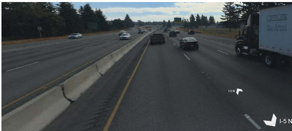
Figure 15. Photo. I-5 cross-section configuration and median barriers after replacement.
