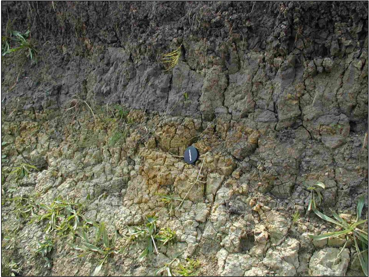
Figure 2.1. Soil cracking due to desiccation at site ST3. Camera lens cap is 5.5 cm in diameter.
