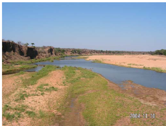
Flood damage is partly caused because of wetland degeneration in the catchment areas
