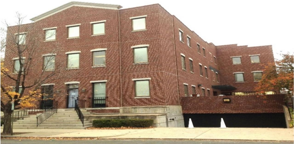
(a). Front view of the building
