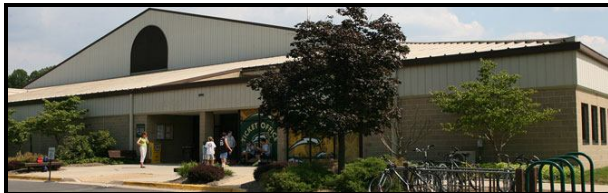
Figure 5.1 George Mason University field house Used with permission ( http://recsports.gmu.edu/files/u1/fieldhouse-exterior-1.jpg )
