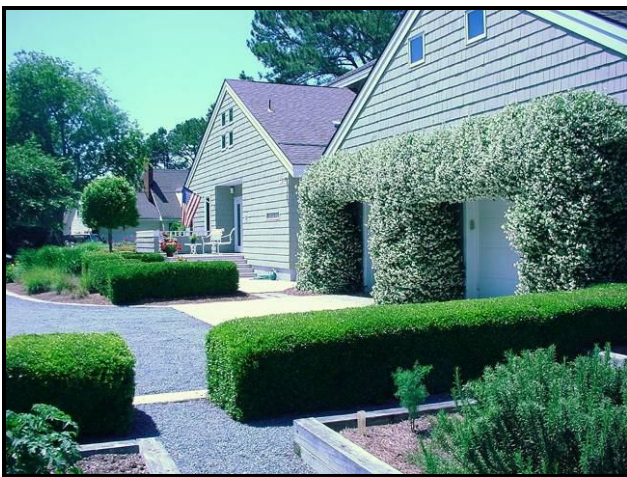
Figure 5.16 Residence B roofline without gutters and downspouts Adrienne J.L. Tucker
