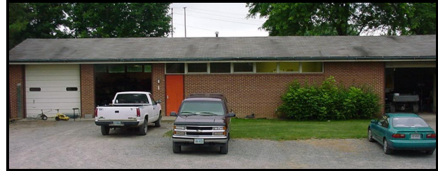
Figure 5.10 Virginia Tech Turfgrass Research Center maintenance building Adrienne J.L. Tucker
