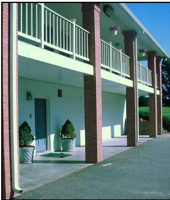
Figure 5.12 Williamsburg Country Club downspouts draining onto the golf path Adrienne J.L. Tucker
