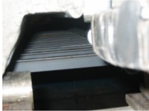
(b) Angle straps underneath the slab
