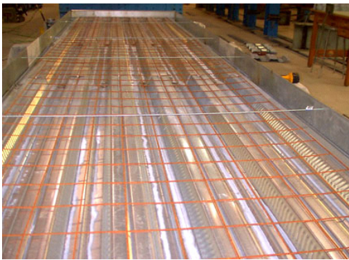
(c) Deck form ready to receive concrete
