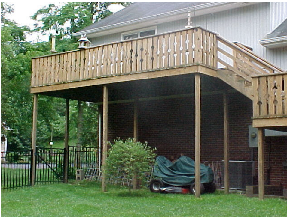
Figure 2- 4. Deck #4 while in-service.
