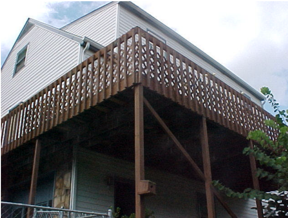
Figure 2- 6. Deck #6 while in-service.
