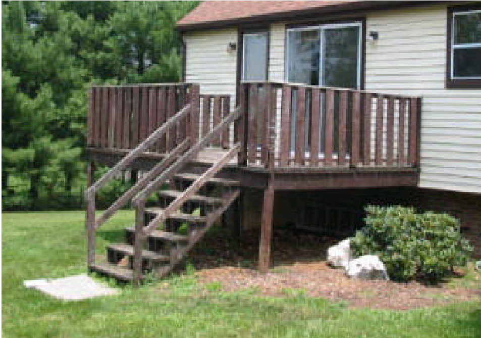
Figure 2- 5. Deck #5 while in-service.
