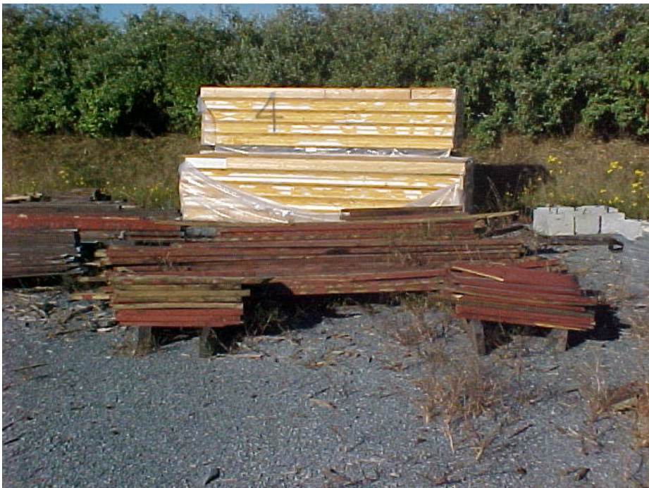
Figure A- 2. Recovered CCA treated wood from Deck #2.
