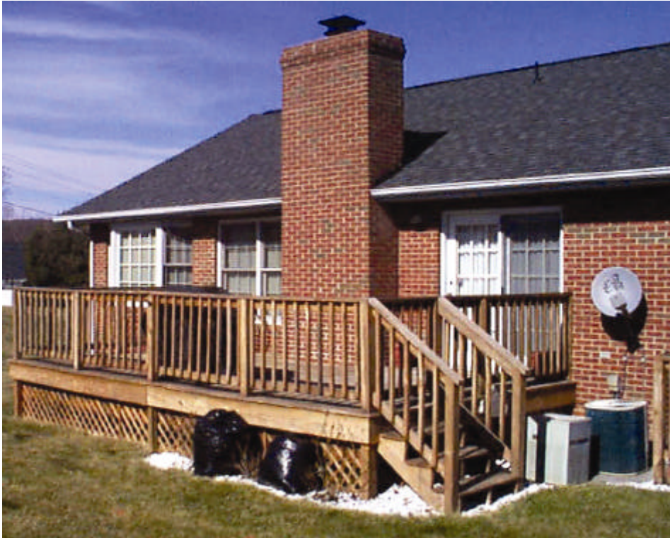
Figure 2- 1. Deck #1 while in-service.
