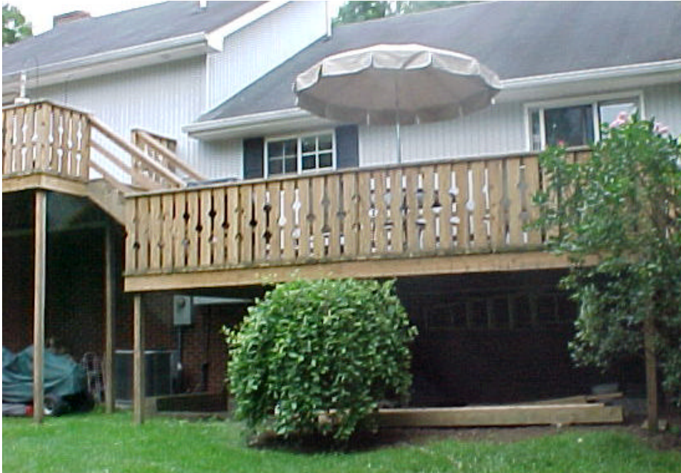
Figure 2- 3. Deck #3 while in-service.
