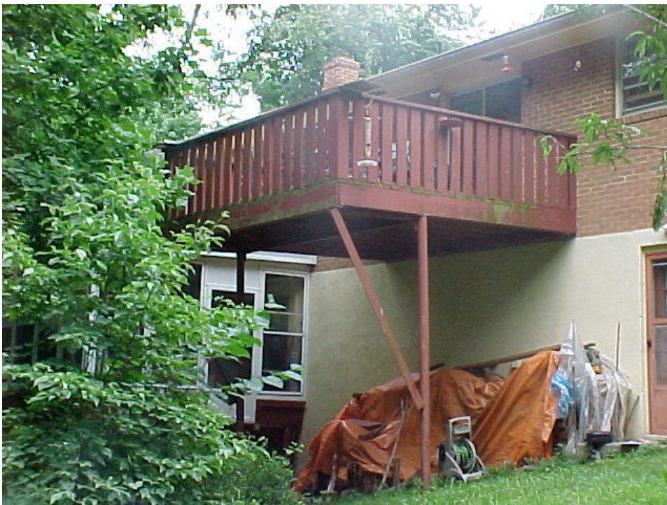
Figure 2- 2. Deck #2 while in-service.
