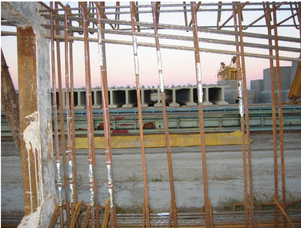
Figure 14. Strain Gages Installed at the 18 ksi Anchorage Zone
