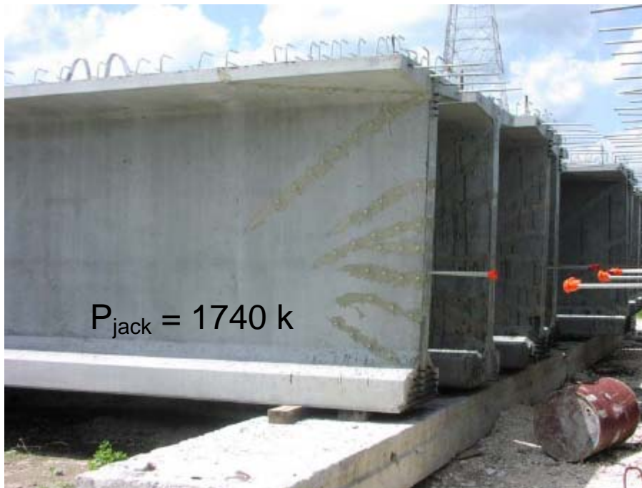
Figure 20. 95.5 in PCBT Beam Ends with Repairs. Photograph from Davis et al. (2005)
