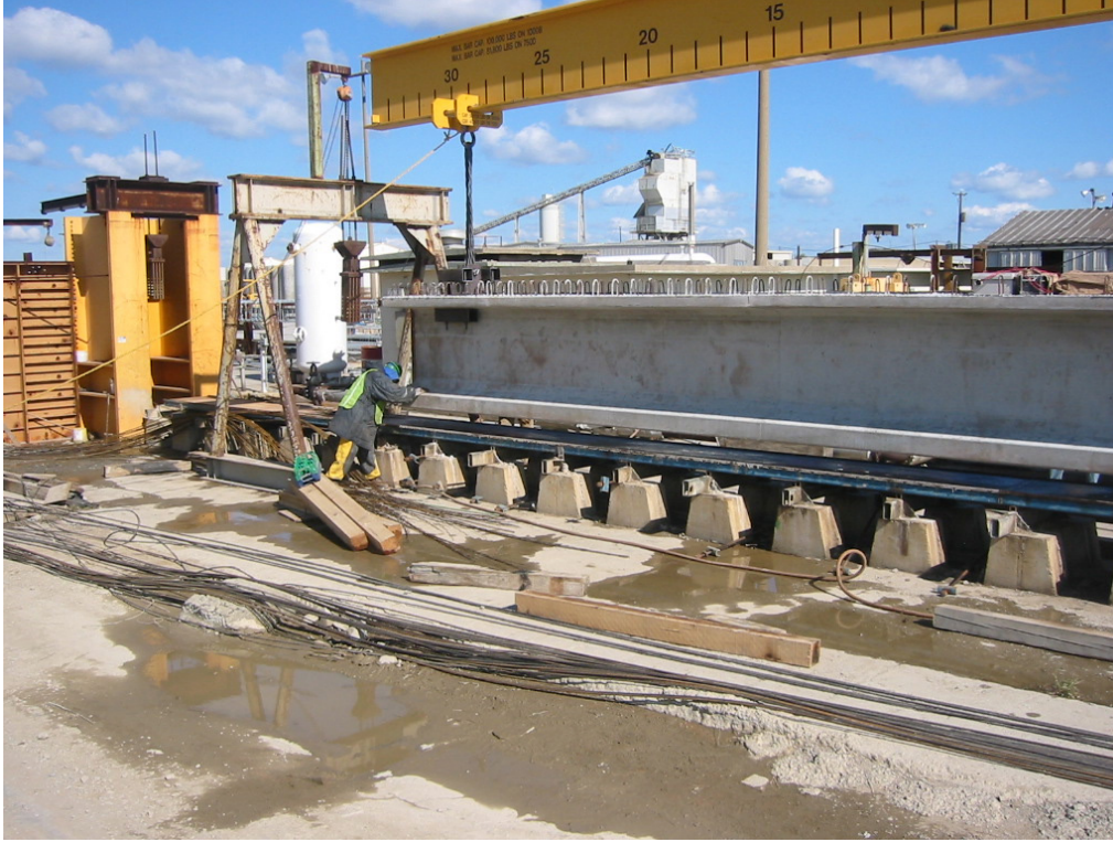
Figure 15. Test Girder Lifted From Casting Bed on October 25, 2006
