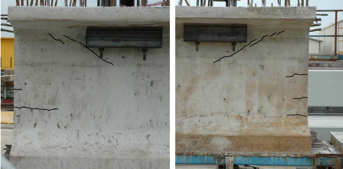
Figure 38. Crack Pattern in the 18 ksi Anchorage Zone After Lifting
