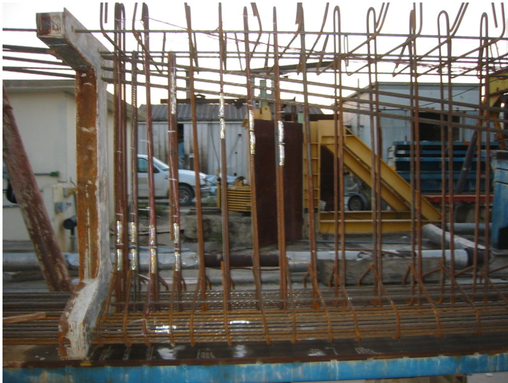
Figure 13. Strain Gages Installed at the 12 ksi Anchorage Zone
