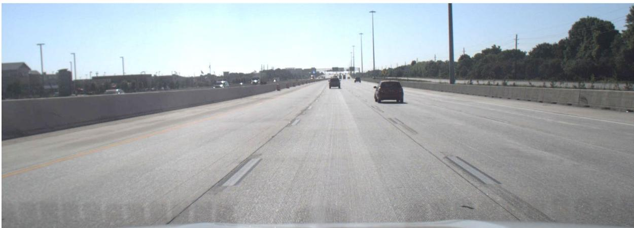
**Figure 20: Image of a road segment with white pavement markings with a black border (driving eastwards).**
