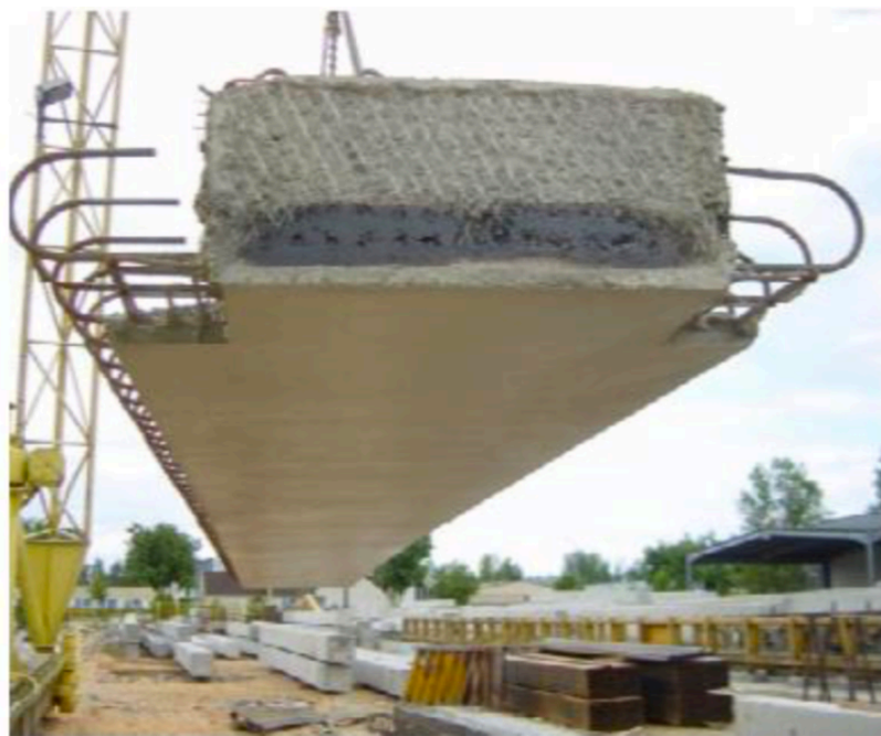
Figure 1-1: Poutre-Dalle system (Bell, 2006)
