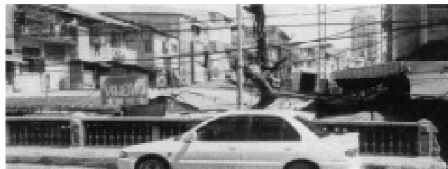
Figure 4.14: The south section of the City Moat Canal is covered by several iron bridges for commercial purposes.
