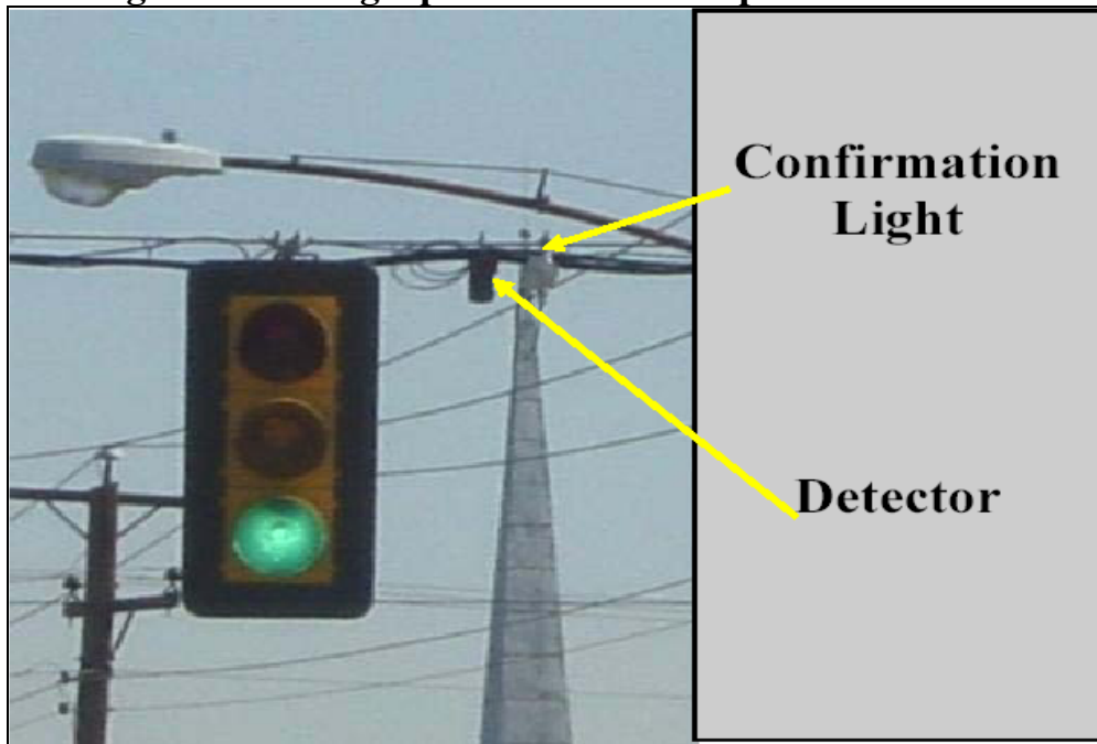
Figure 8. Photographs to show 3M Opticom Emitters
