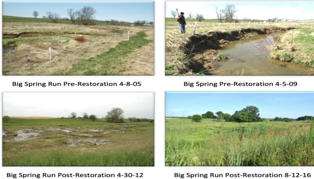
Figure 8. Pre- and post-restoration images of a legacy sediment removal stream restoration near Lancaster, Pennsylvania (Sep-Nov, 2011). The pre-restoration stream length was 2,731 ft and after, 2,960 ft. Restoration design and figure adapted from LandStudies, Inc., Lititz, PA.
