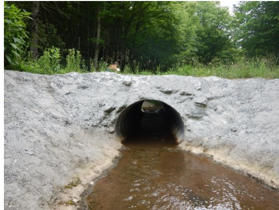
Figure 10. Jackson Fork 2 road crossing, downstream view.
