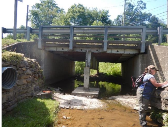
Figure 2. Big Lick Creek 1 road crossing, downstream view.
