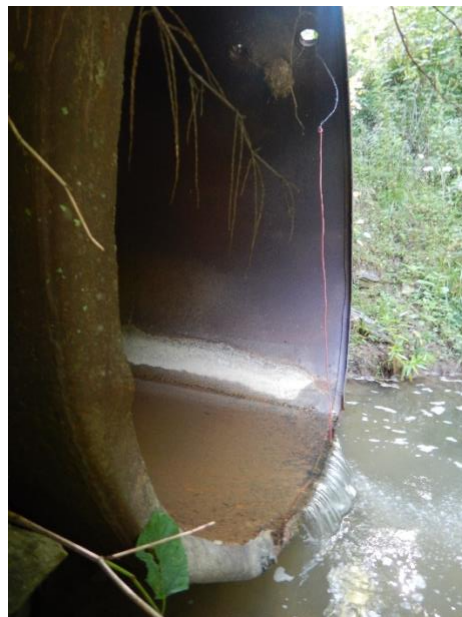
Figure 7. Hart Creek 2 road crossing, downstream view.
