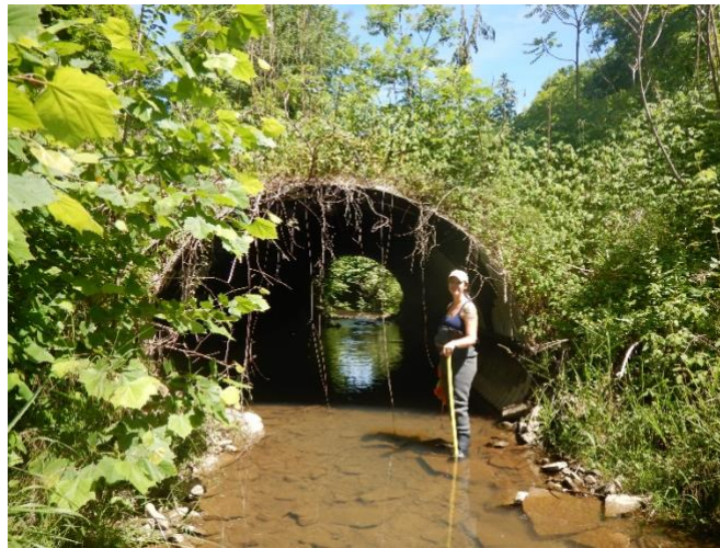
Figure 12. Lewis Creek 3 road crossing, downstream view.
