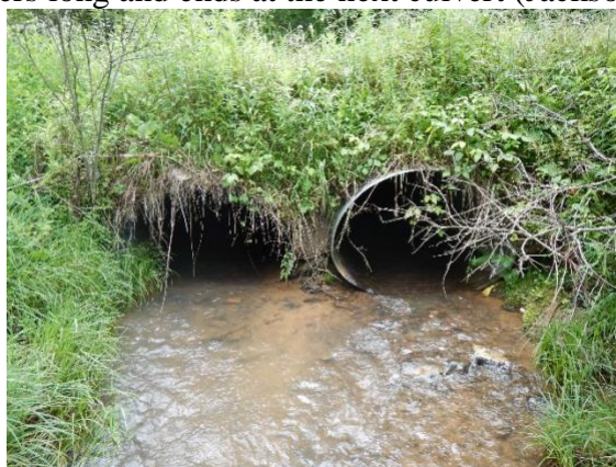
Figure 9. Jackson Fork 1 road crossing, downstream view.
