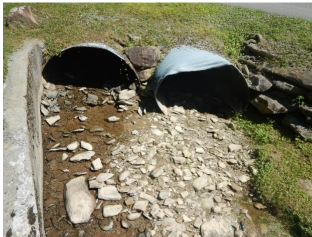
Figure 3. Big Lick Creek 2 road crossing, downstream view.
