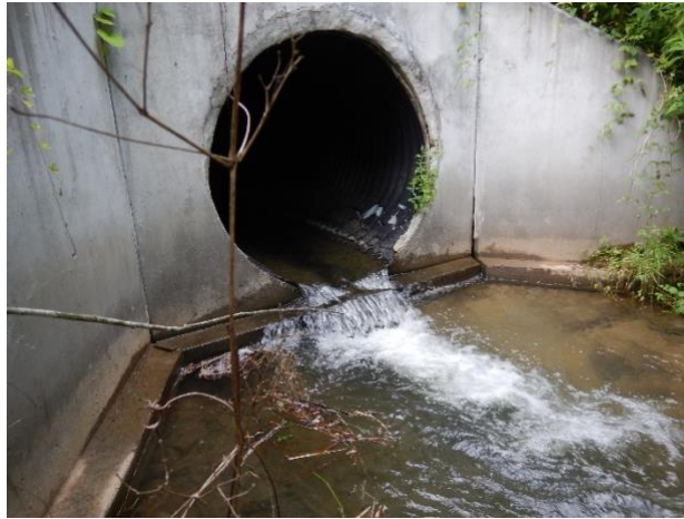
Figure 14. Middle Creek 3 road crossing, downstream view.
