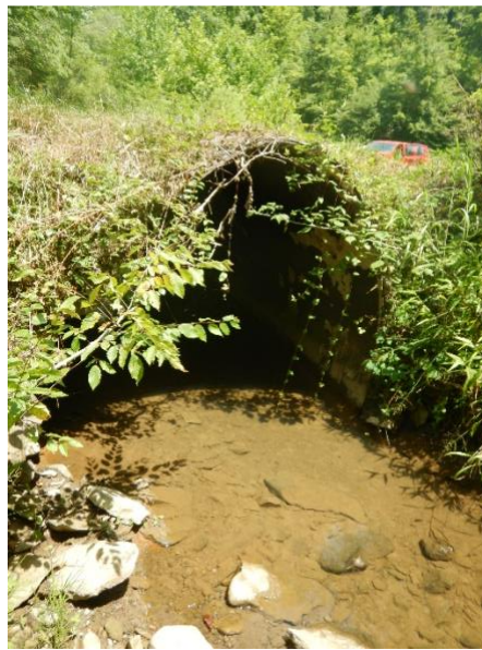
Figure 4. Big Lick Creek road crossing, downstream view.
