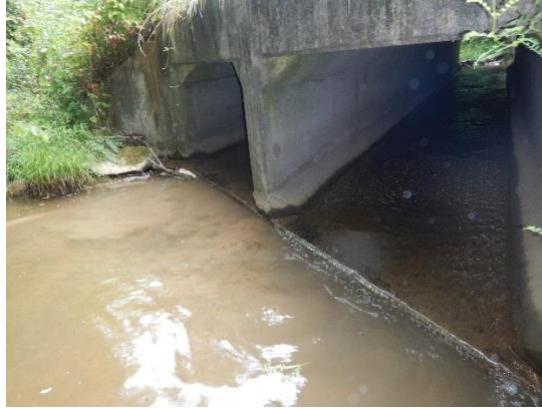
Figure 6. Hart Creek 1 road crossing, downstream view.
