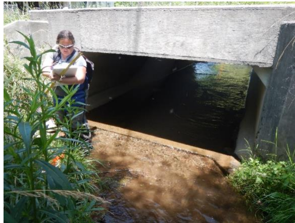
Figure 13. Lewis Creek 4 road crossing, downstream view.
