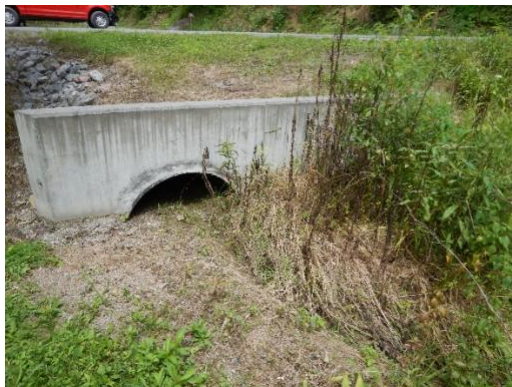
Figure 8. Hess Creek 2 road crossing, downstream view.
