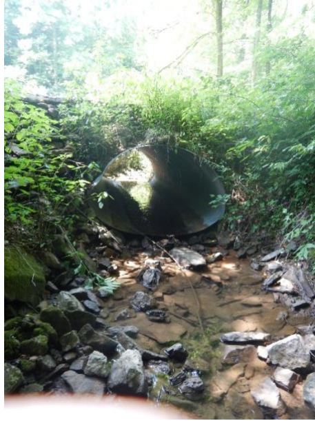
Figure 5. Big Lick Creek 4 road crossing, downstream view.
